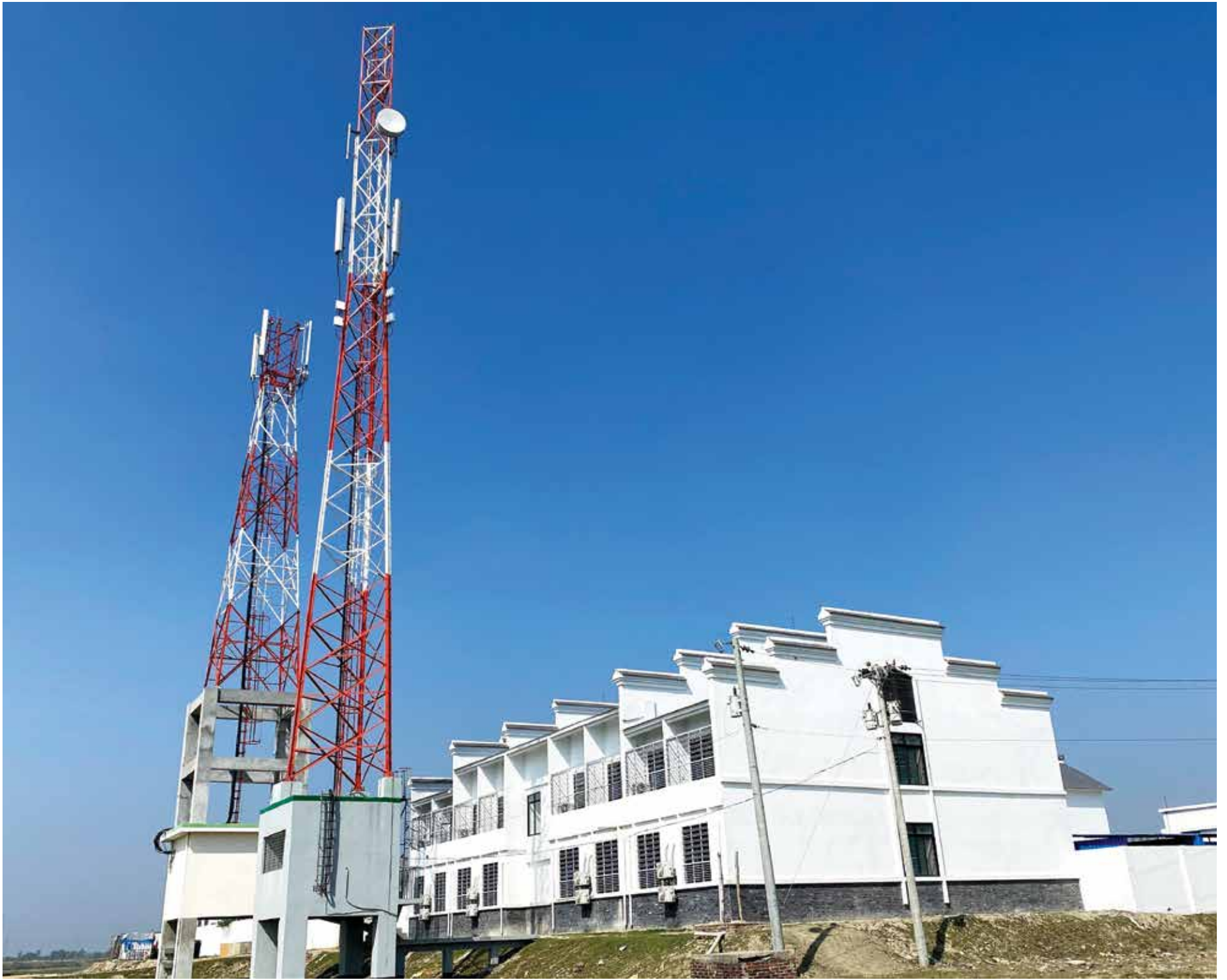
Telecommunication Tower at Banagabandhu Shilpanagar.
