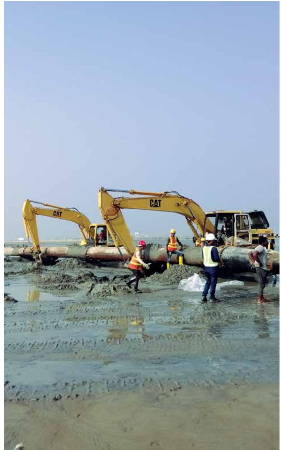
Land development works to serve investors.
