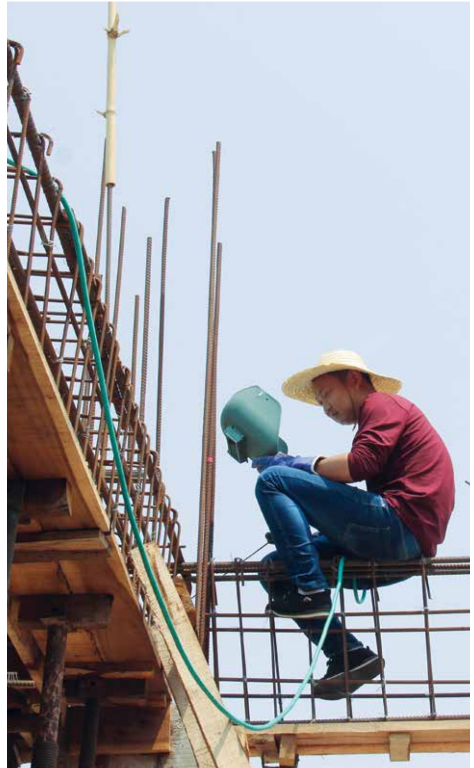
Construction works of a building inside BSMSN.
