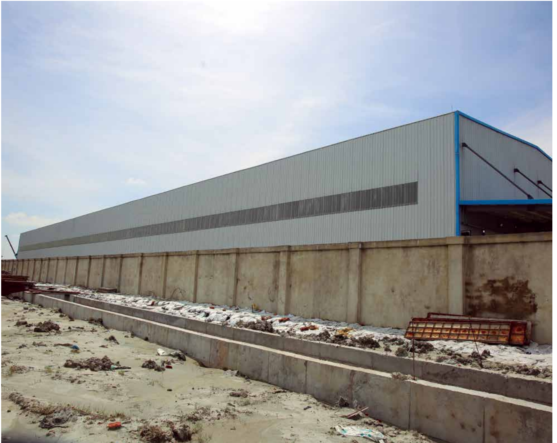
Construction of a 100% export oriented chemical industry Jinyuan Chemical Co. Ltd.
