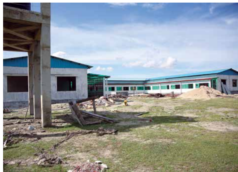
Undergoing building works of security shed for the industrial city.
