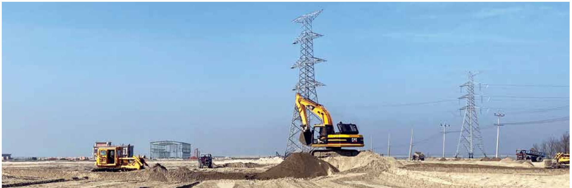
Land development at Bangabandhu Shilpanagar.
