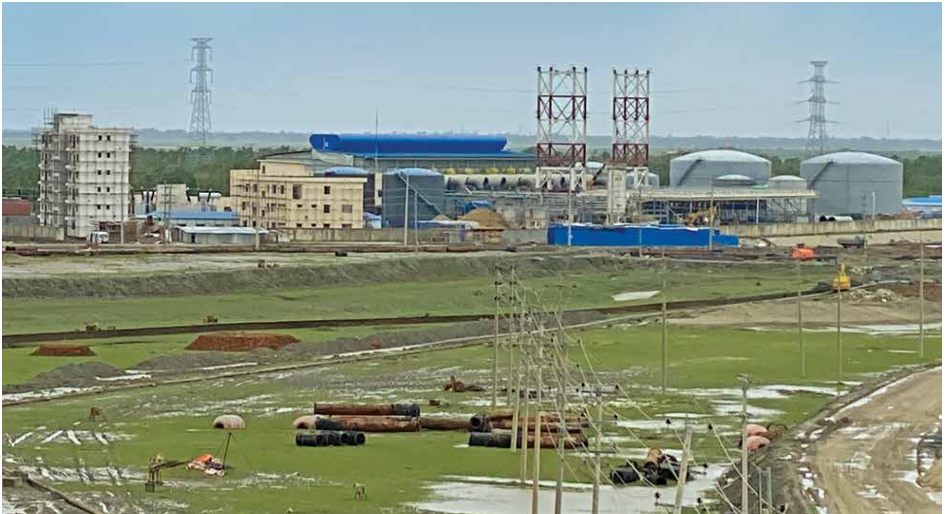
A 150 MW power plant at Bangabandhu Sheikh Mujib Shilpanagar.
