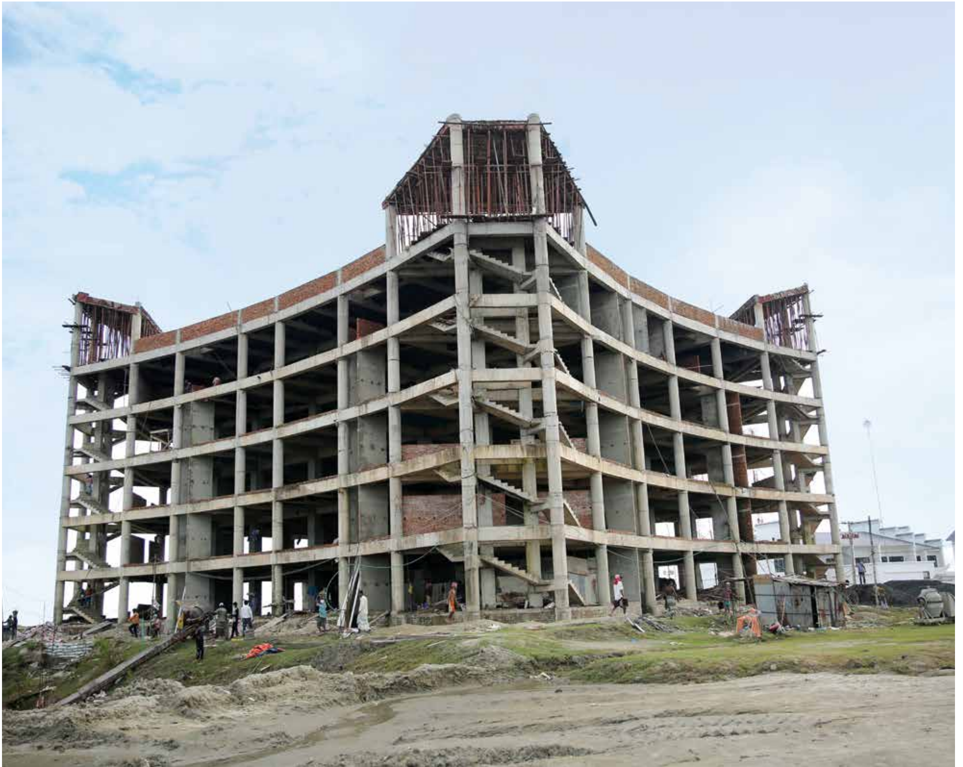
Construction of administrative building of BSMSN is under way.
