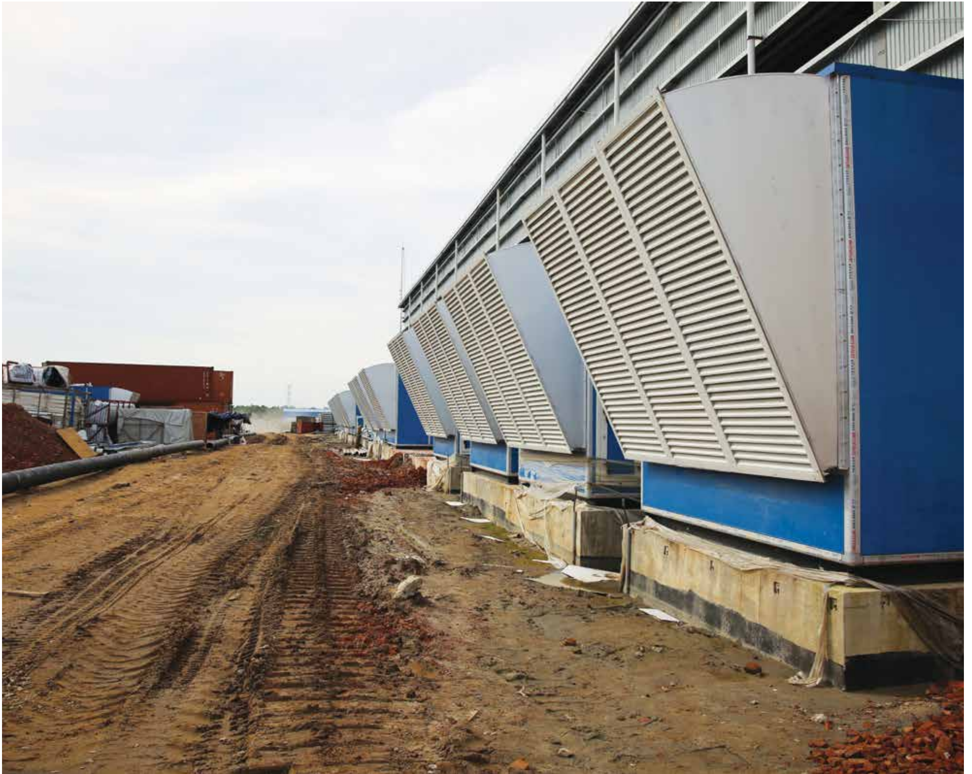
Ongoing construction works at Bangabandhu Sheikh Mujib Shilpanagar.
