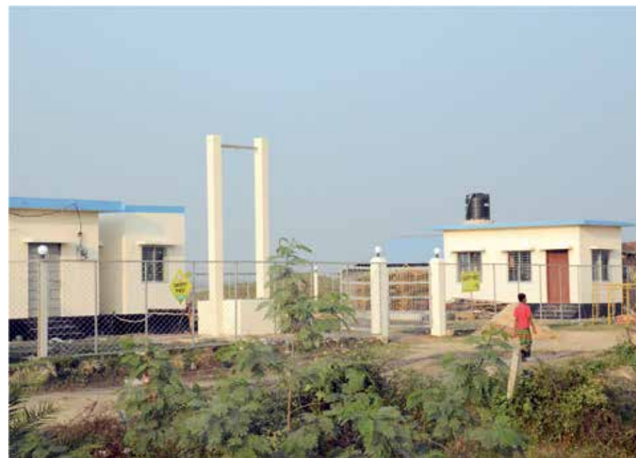
A water pump inside Bangabandhu Sheikh Mujib Shilpanagar.
