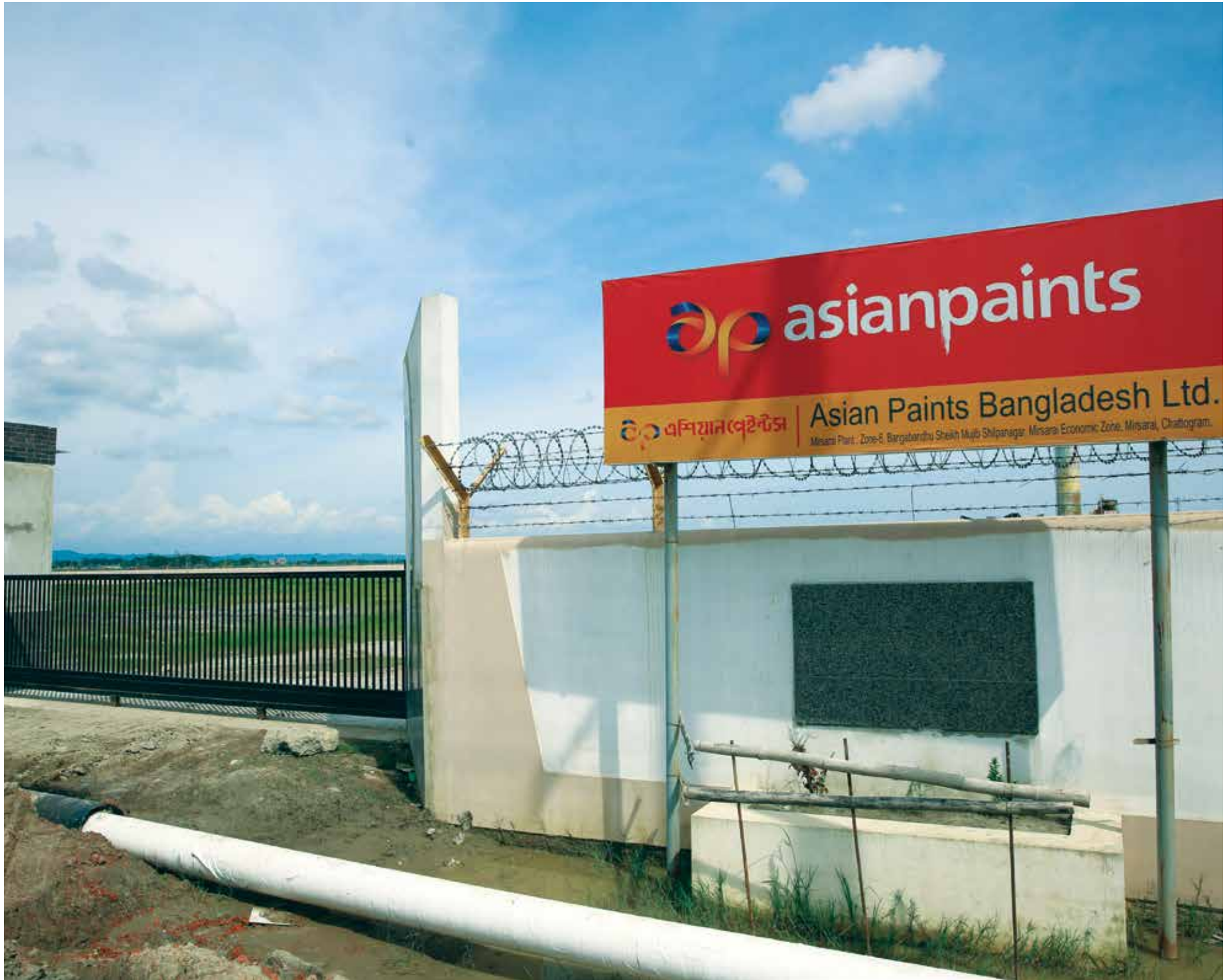
Undergoing construction work of Asian Paints factory.
