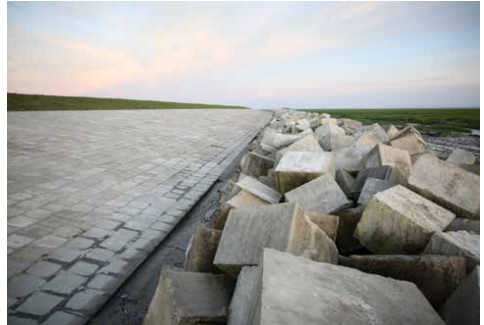
22 kilometre long superdyke is being built along the Bangabandhu Shilpanagar.
