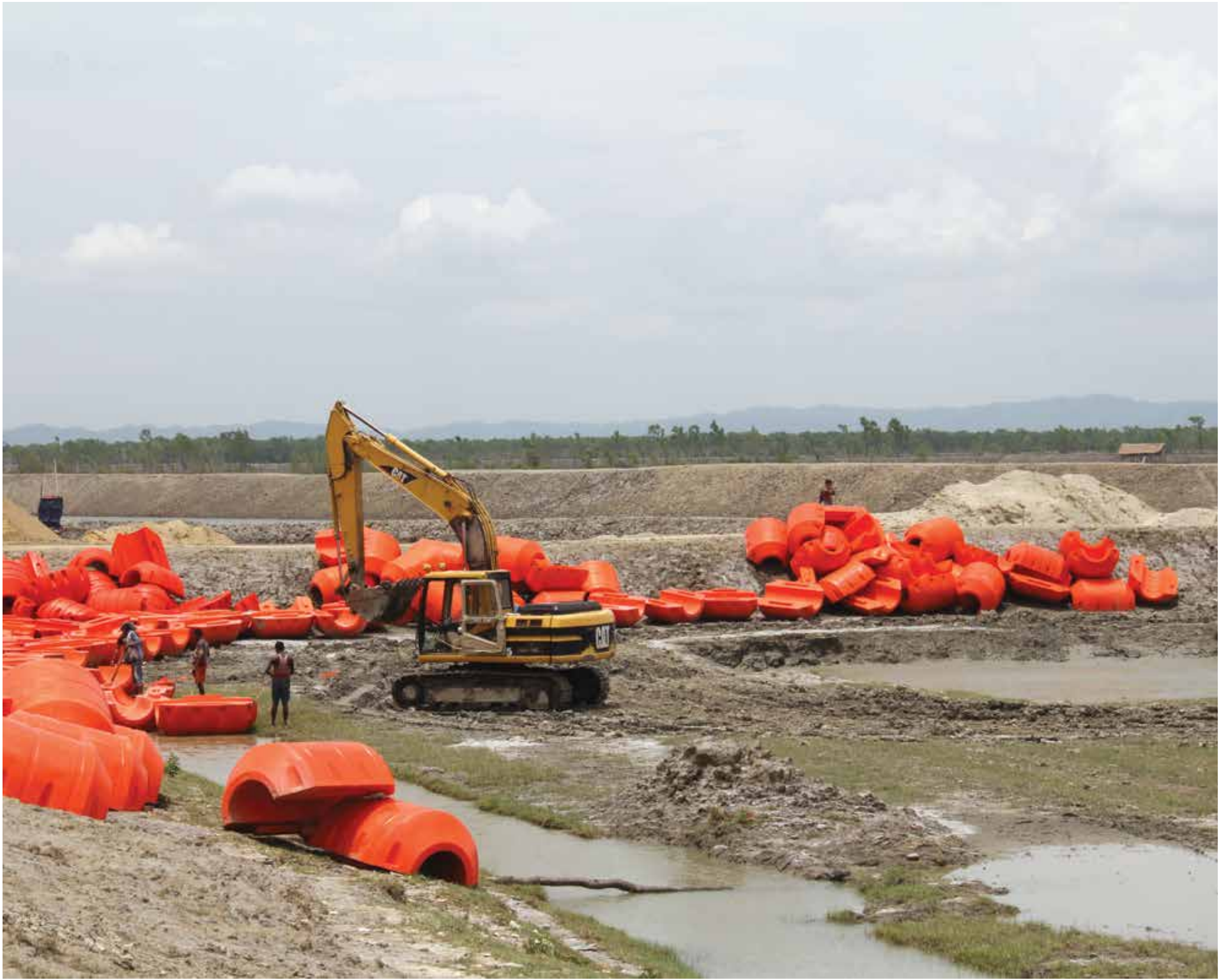
Earthworks being carried out to develop industrial plots inside the zone.
