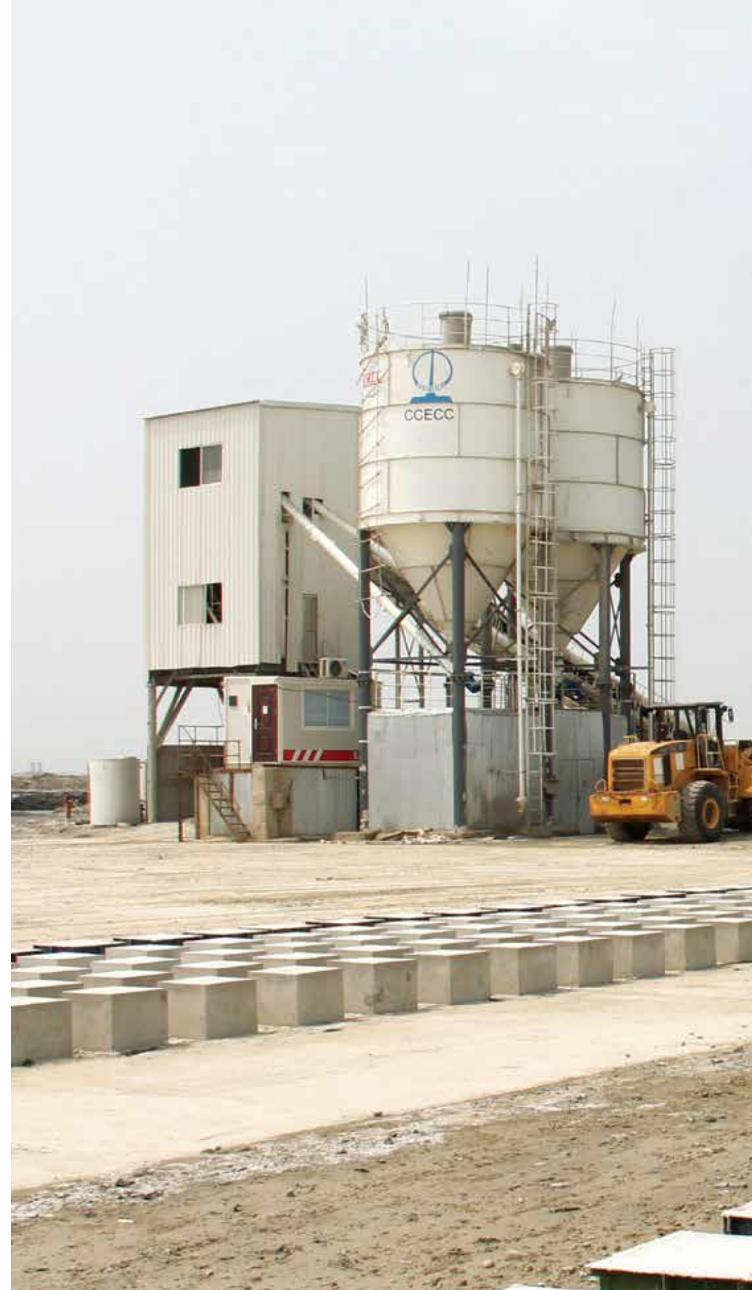
A yard dedicated to building concrete blocks for the superdyke.
