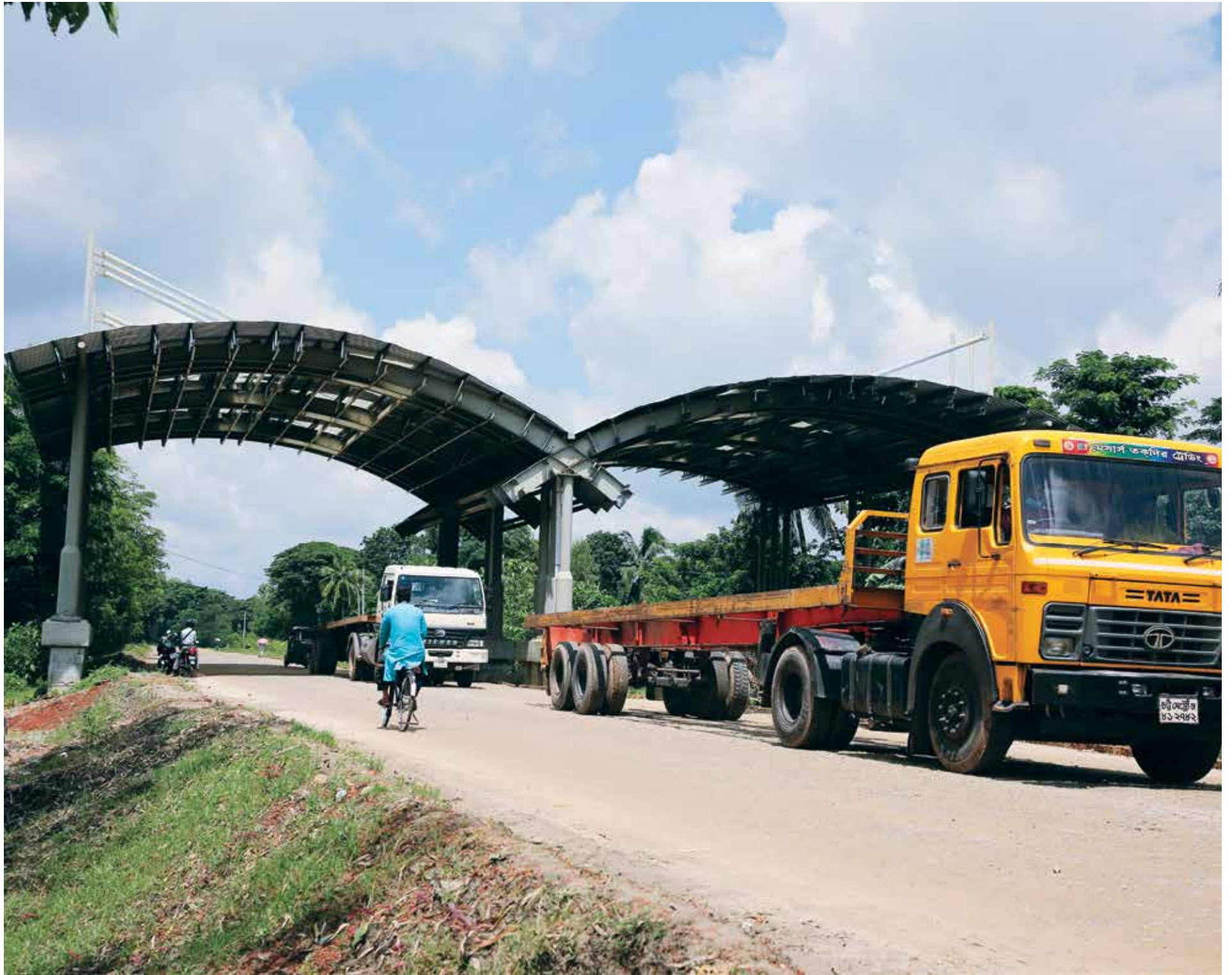
Construction of entry gate for Sheikh Hasina Avenue.
