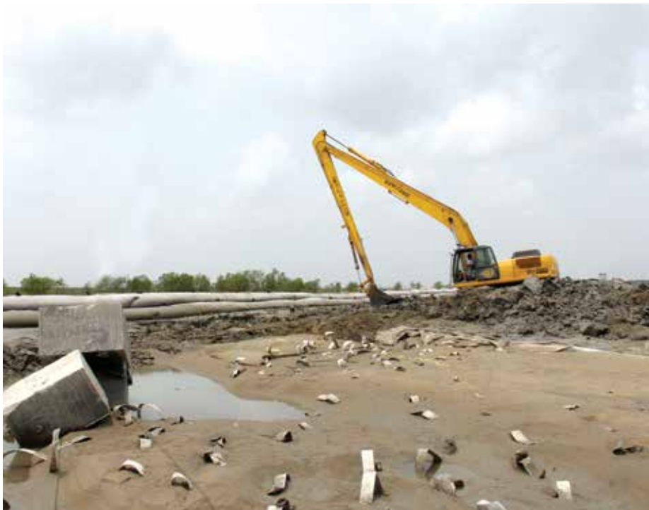
Soft soil improvement works with pre-fabricated vertical drains is under way.
