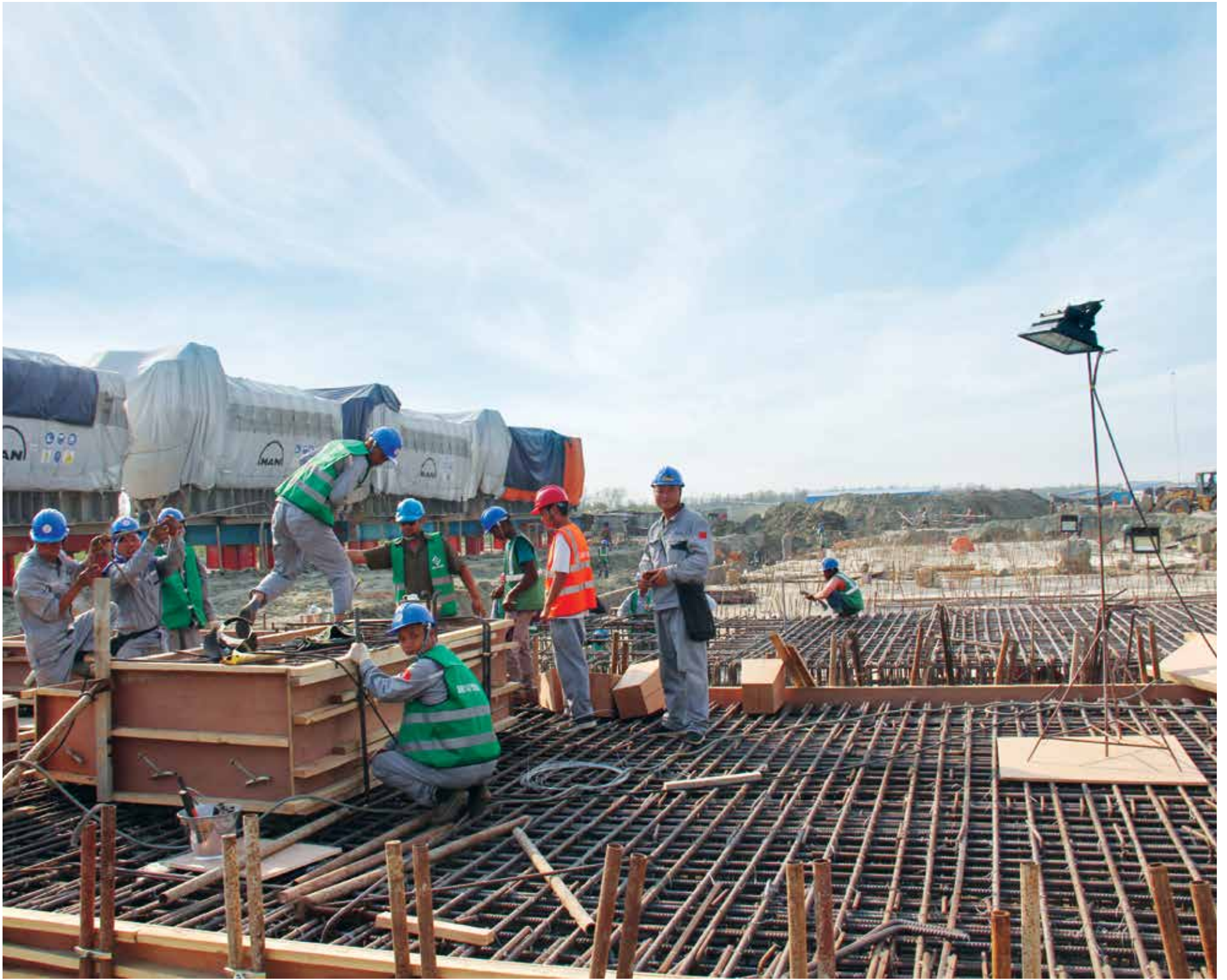
Workers busy at work.
