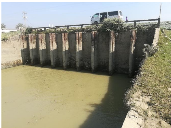
Figure 2.15: 9 vent regulator of Ichakhali khal
