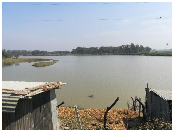
Figure 2.16: Reservoir at Ichakhali khal regulator site
