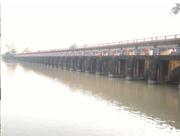
Figure 2.19: 40 vent regulator on Feni River
