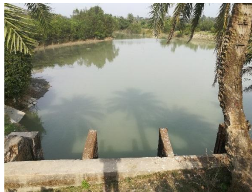
Figure 2.5: Upstream of Shaherkhali khal at regulator site
