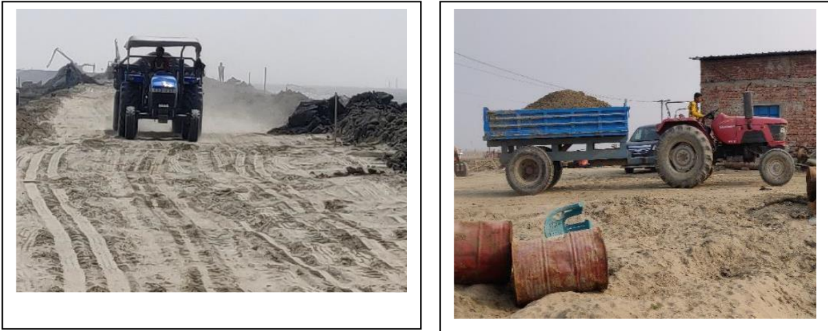
Photo 6-1: Ongoing work at PSDSP site
