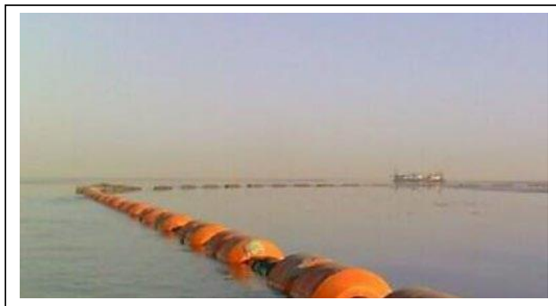
Photo-9-2: Pipe line for transporting dredged material
