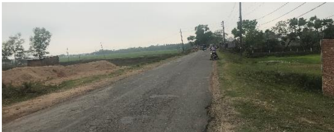
Figure 10-2: Netrokona-Mohonganj Road (Front side road of proposed area)
