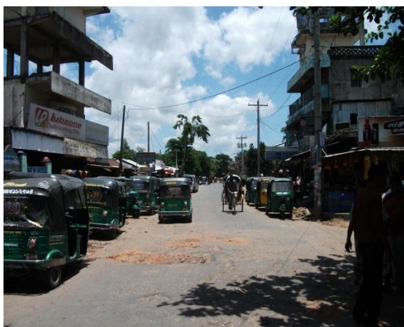
View of access road -i (DC Obaidullah Road) from Dhaka-Chittagong old Highway (Borotakia Bazar intersection point) leading to BWDB Embankment at Noapara in Roypur Union, Mirershorai Project site at southern part.
