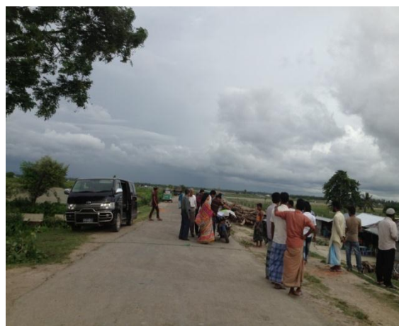
View of Muhuri Project Embankment near Regulator (behind) at intersection of Feni River and Embankment with CDSP Embankment joining to the Muhuri Project Embankment ahead.
