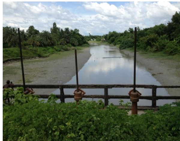
Sluice gate in BamonSundor village near coastal forest
