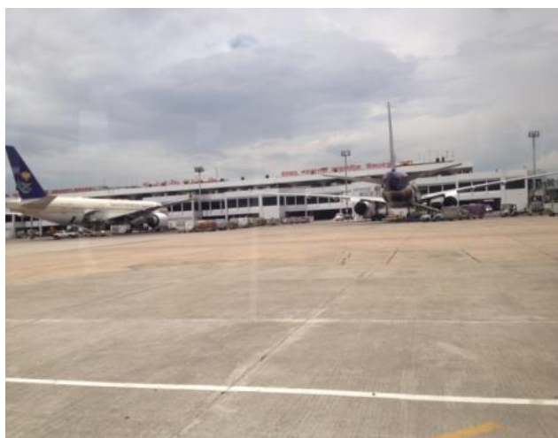
Chittagong International Airport
