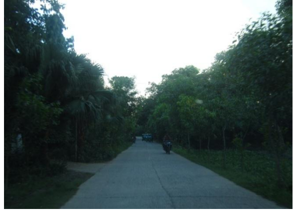
View of access road - i (DC Obaidullah Road) as seen on the way to site.
