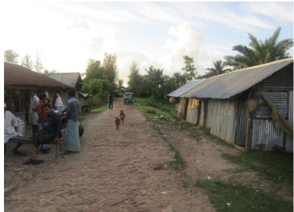
View of BWDB main Embankment as seen from Embankment-DC Obaidulla Road Intersection towards Baman Sunder Forest area to the north.
