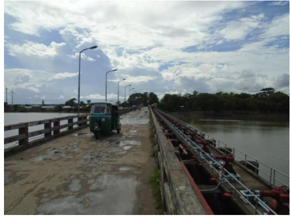
Muhuri Dam (Sluice Gate) on Feni river
