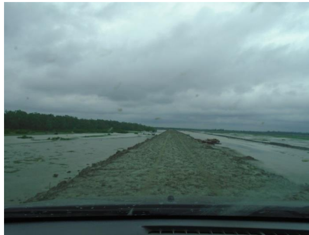
View of access road for Mirsarai 2B portion to main access road
