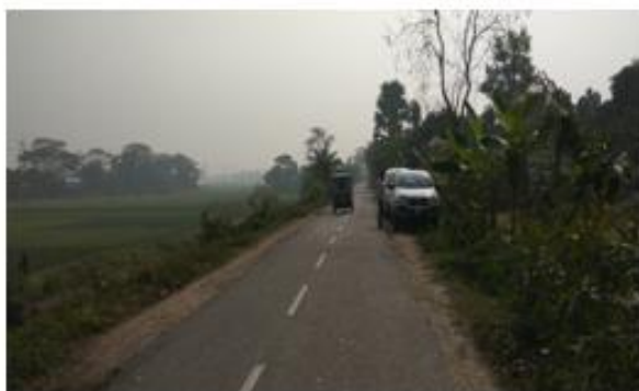
Road along eastern boundary of the EZ site
