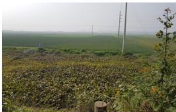
Power transmission line passing through EZ site
