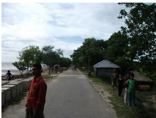
Another view of Embankment towards project site with Paved road on top.
