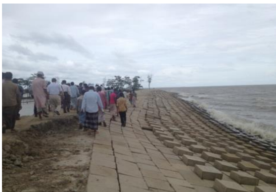
Status of dikes and road on top leading to the tip of the Peninsula
