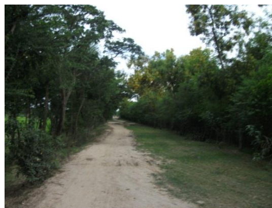
View of BWDB Embankment with earthen road top. Stable side slope with tree plantation is seen in the view.
