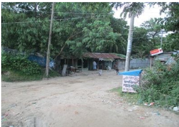
Another view of 2 nd access road as seen from the BWDB Embankment near the EZ site. The road runs towards north-east (about 8km) till it meets the Chaturi Bazar-CUFL road at Bandar Centre.
