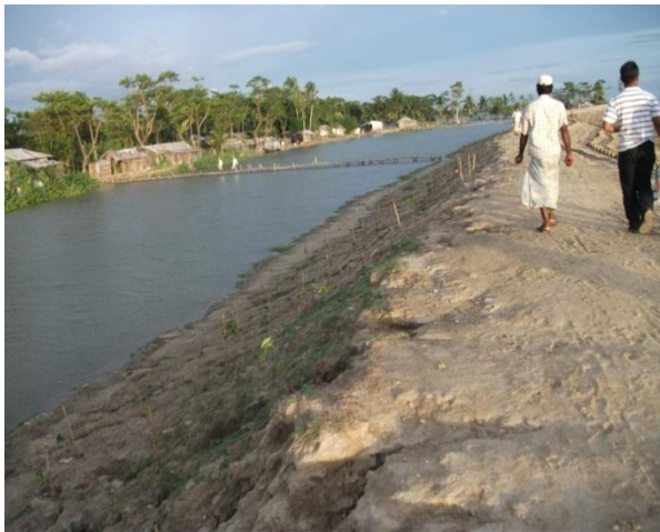
View of EZ site along the BWDB Embankment.
