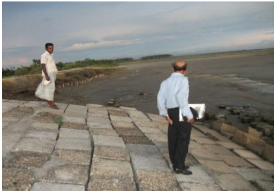
View of char near Sangu River as seen from the Embankment.
