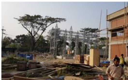
Substation under construction at Solakhali
