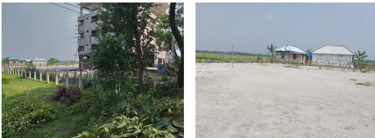
Figure 78: Newly Constructed building in the proposed Gopalganj site
