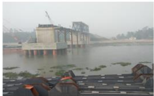
Single track railway line under construction towards Gopalganj
