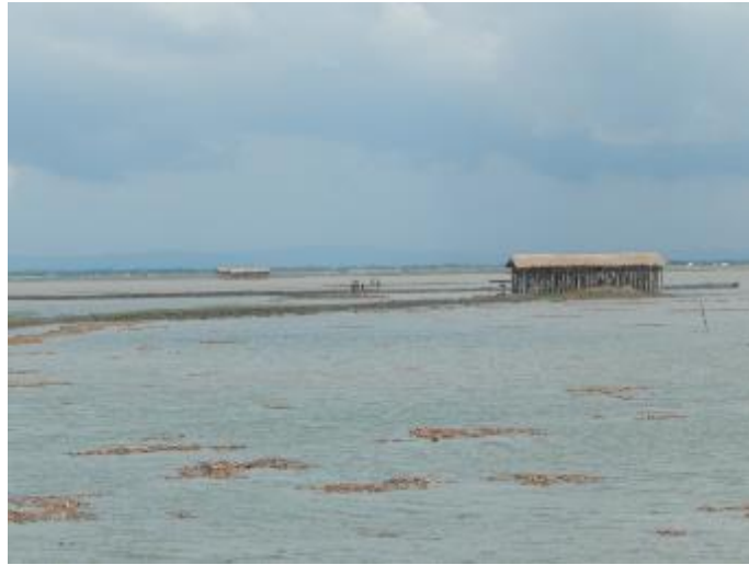
Figure 39: Water Logged in the Project Area due to Tidal Flood
