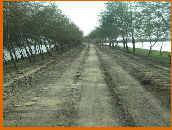
Under Development Access Road on BWDB Bund
