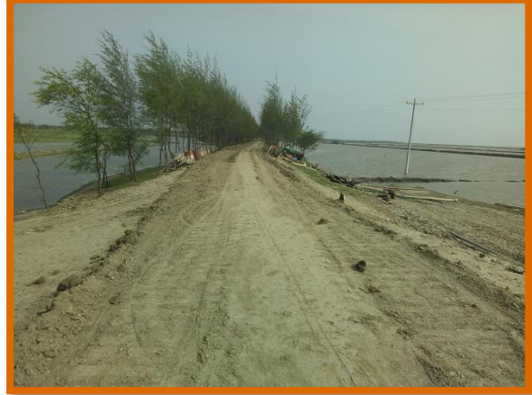
Under Development Access Road on CDSP Bund
