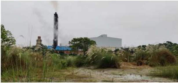
Power plant adjacent to the site
