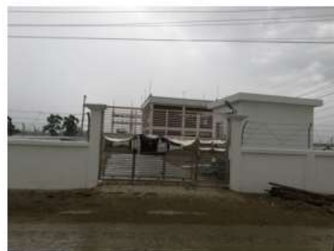
Nearest sub-station of 20 MV capacity at Tikorpur
