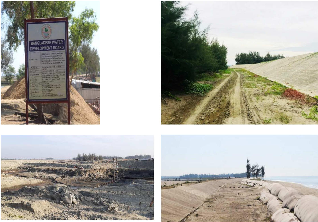
Figure 3-1: Construction of Super dyke of Sabrang Tourism Park
