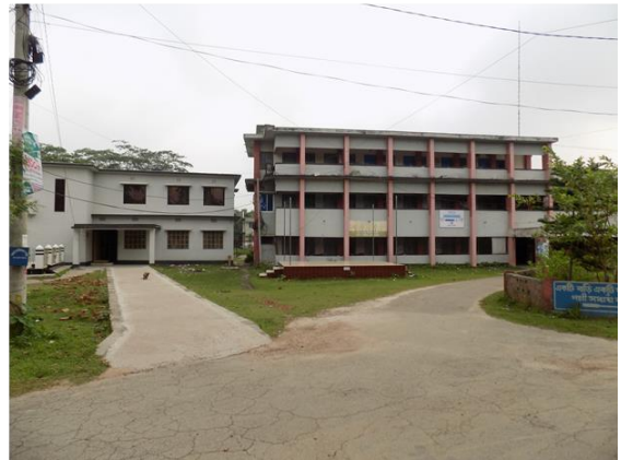
Agailjhara upazila roads
