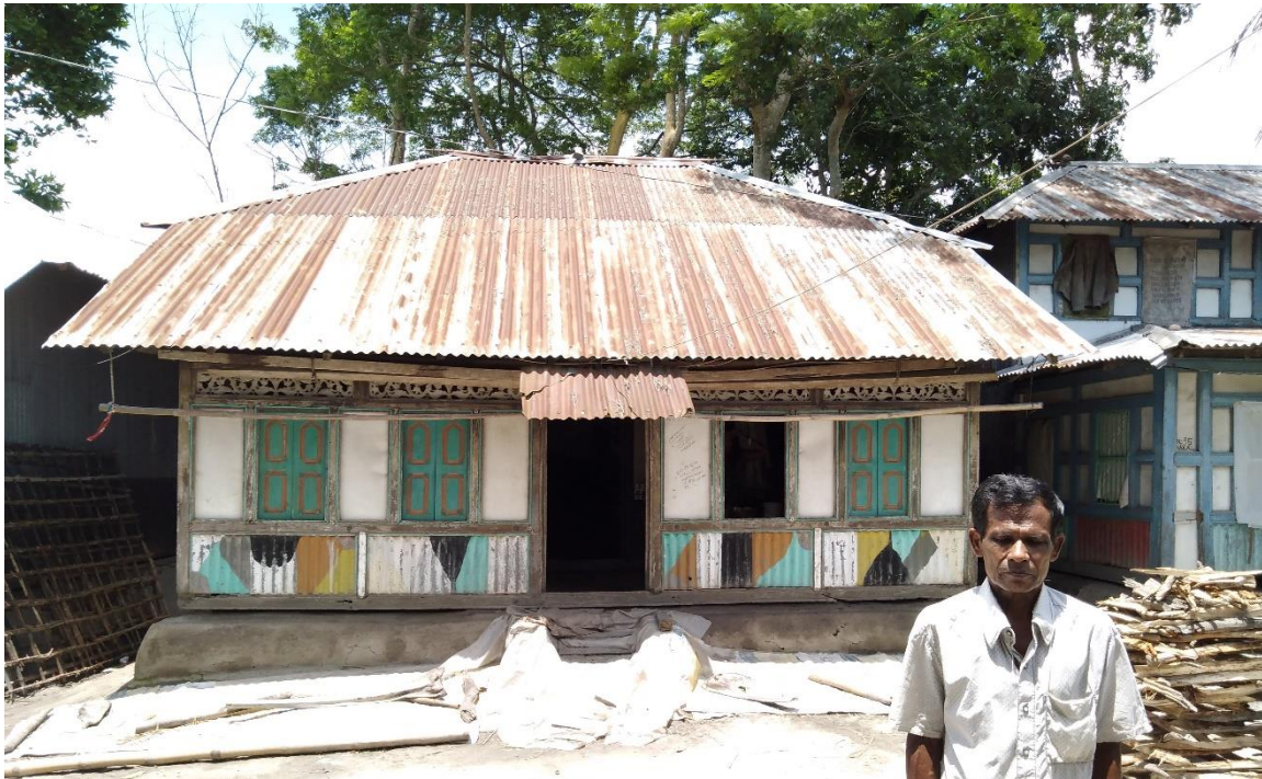
Figure 84: A typical housing structure in project area
