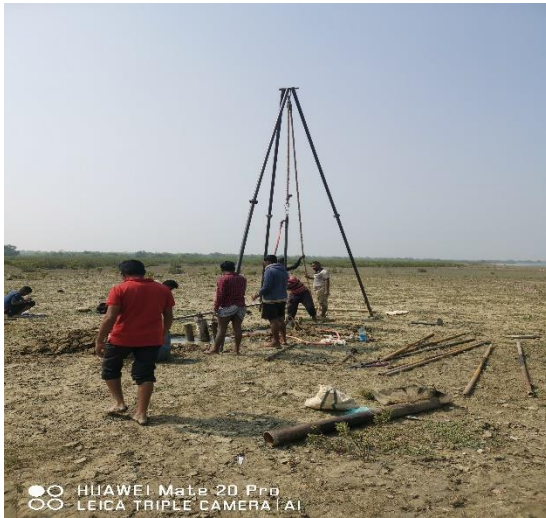
Exploratory boring operation at proposed site BH-2 ( 21^{\circ}29'55.61''\text{N} , 91^{\circ}52'59.62''\text{E} )
