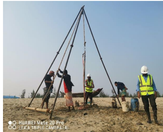
Exploratory boring operation at proposed site BH-5 ( 21^{\circ}28'50.99''\text{N} , 91^{\circ}55'27.45''\text{E} )
