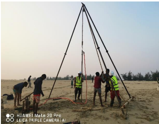
Exploratory boring operation at proposed site BH-6 ( 21^{\circ}28'39.28''\text{N} , 91^{\circ}54'35.93''\text{E} )
