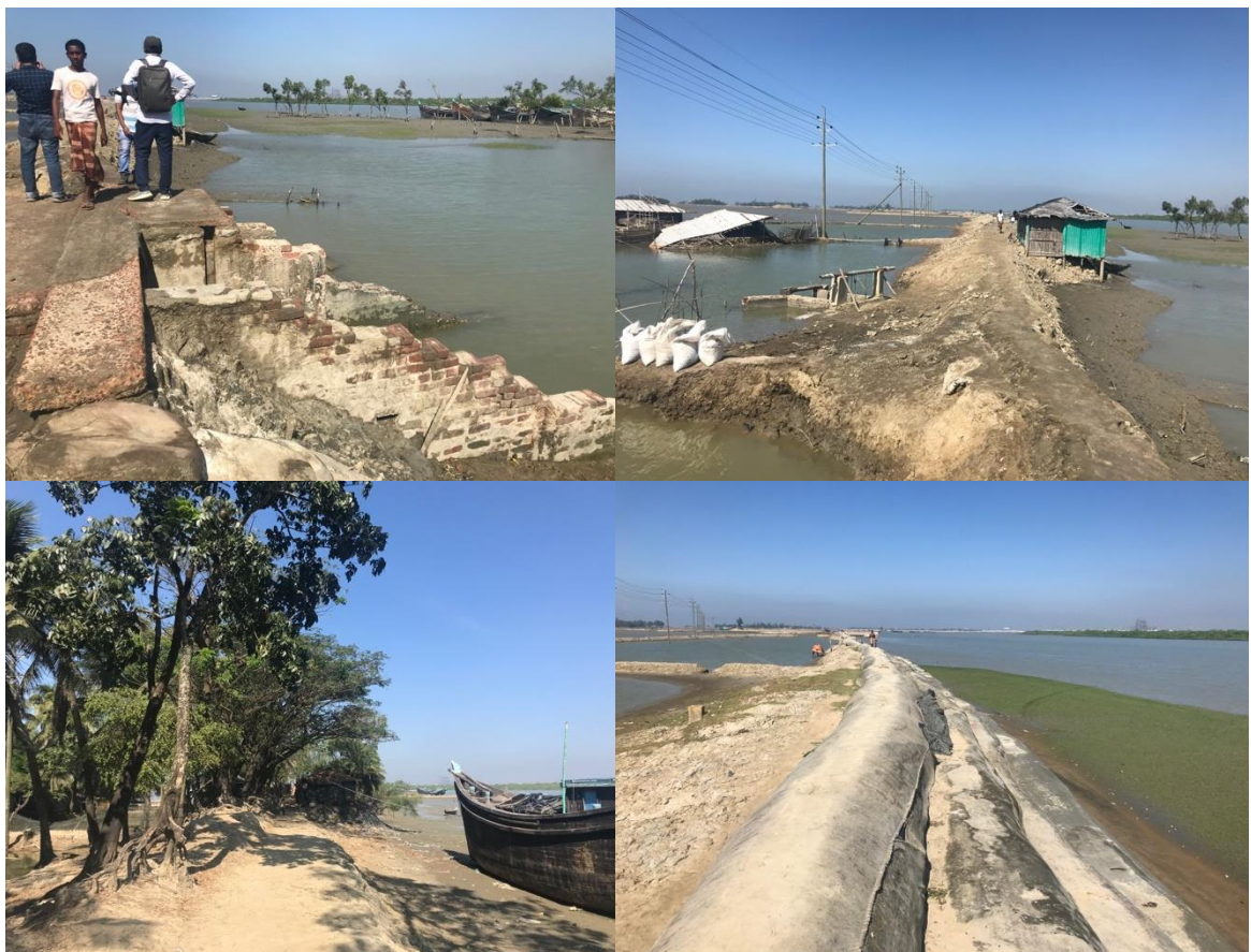
Figure 4.7: Existing Condition of the Embankment
