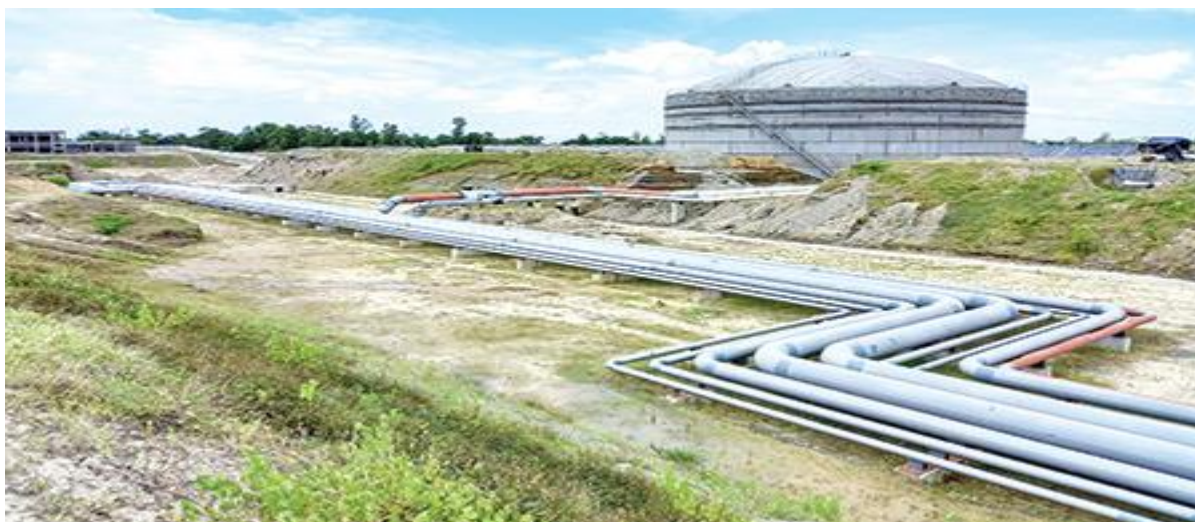
Figure 2.7: SPM Pipeline Project
