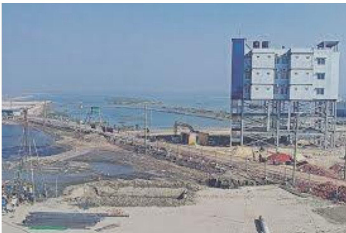
Figure 2.4: Matarbari 1200 MW Coal Based Power Plant Site under Construction
