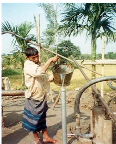
Figure M.5: Monitoring well hydraulic connectivity test
