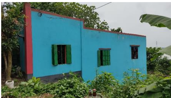
Pucca House in the Approach Road Alignment
