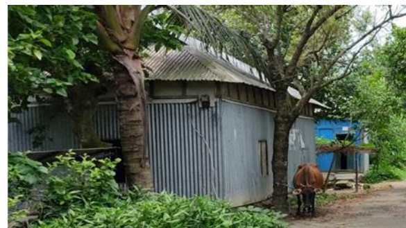
Kutcha House in the Approach Road Alignment
